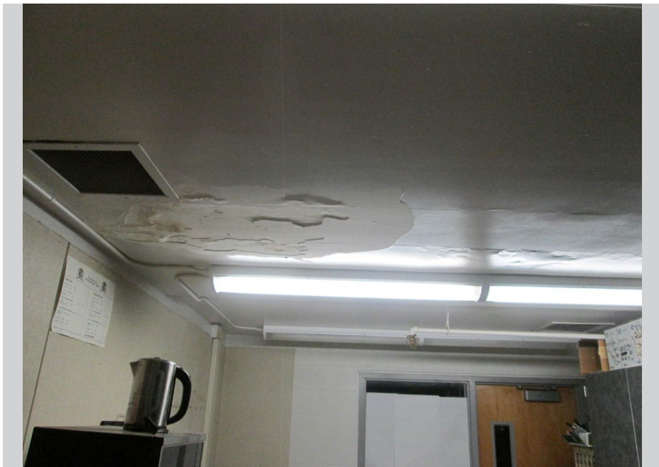
Ceiling damage - requires repair/replacement
