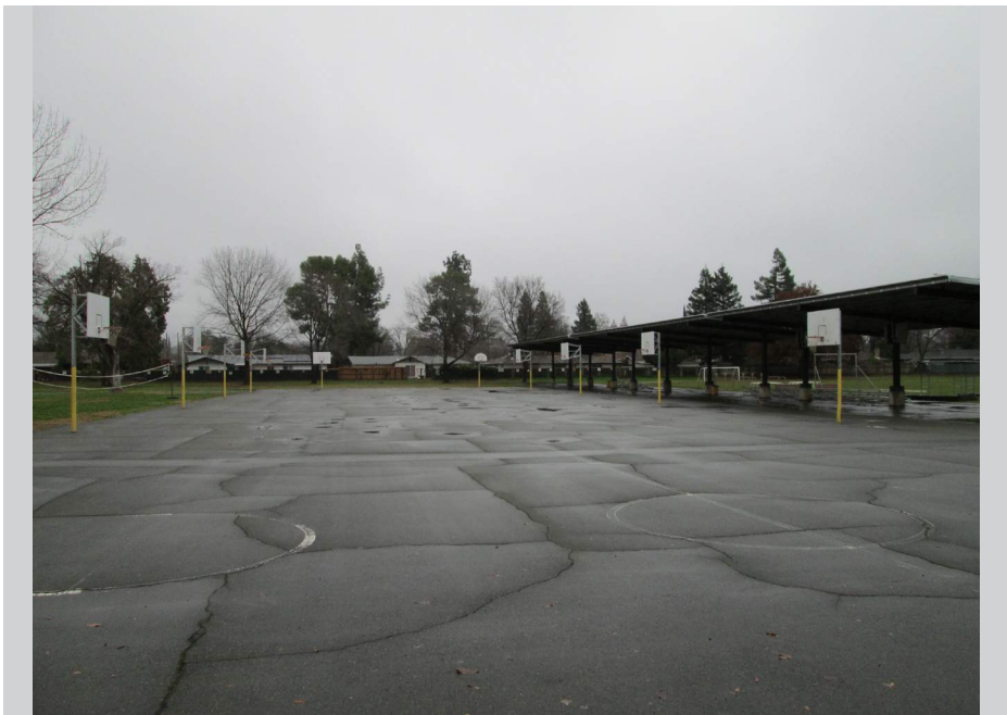
cracking asphalt in need of repair
