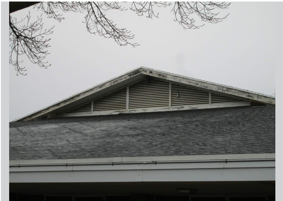
Fascia repair/repaint improvements required
