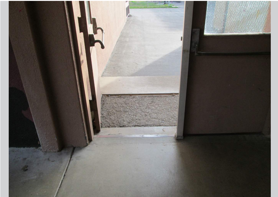
Door thresholds and landings ADA improvements required
