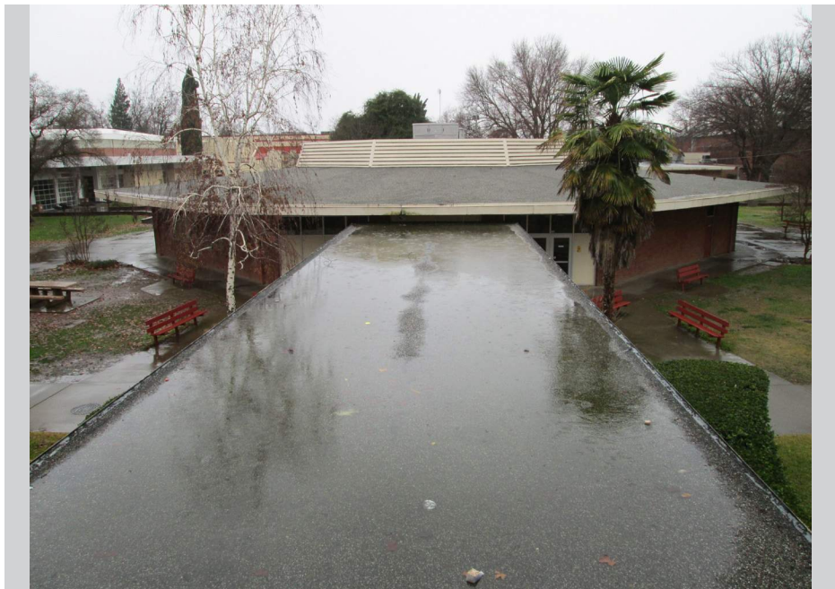
Roof drainage improvements for puddling at covered walkways
